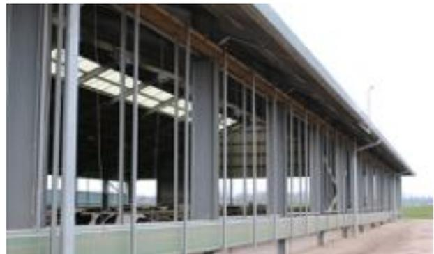
Adjustable gale breakers to ensure the building is optimally ventilated in all weather conditions
